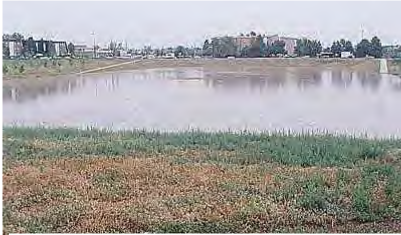
Iloff Stormwater Detention Basin on Goldsmith Gulch
