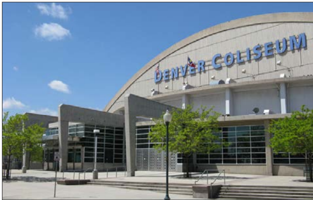
The Denver Coliseum is a potential facility for reuse to support the NWC.
