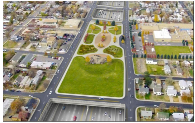
The I-70 East project will be reconstructed between Brighton Boulevard and Colorado Boulevard with a lowered segment of the highway. A new covered park is proposed at Swansea School.
